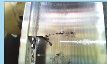
Defect on tread
